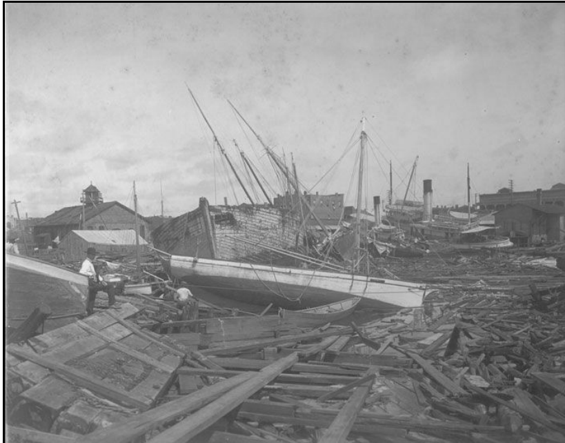
Damaged wharf at Pensacola Florida just after the 1906 hurricane.
